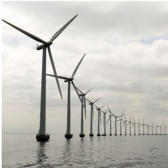
A view of the Middelgrunden offshore wind farm in Denmark consisting of 20 turbines (UN Photo/Eskinder Debebe)
